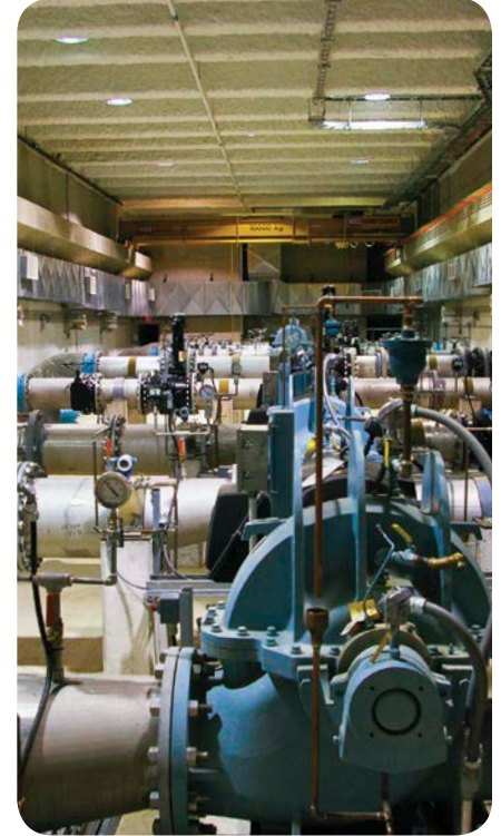
Eramosa designed and programmed the automated control system for this water pumping station capable of pumping over 900L/s of potable water for one of Ontario’s largest municipalities.
